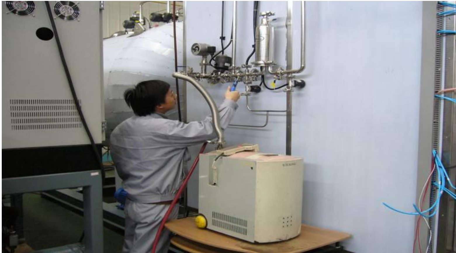
Helium Leak Detector For leakage test
